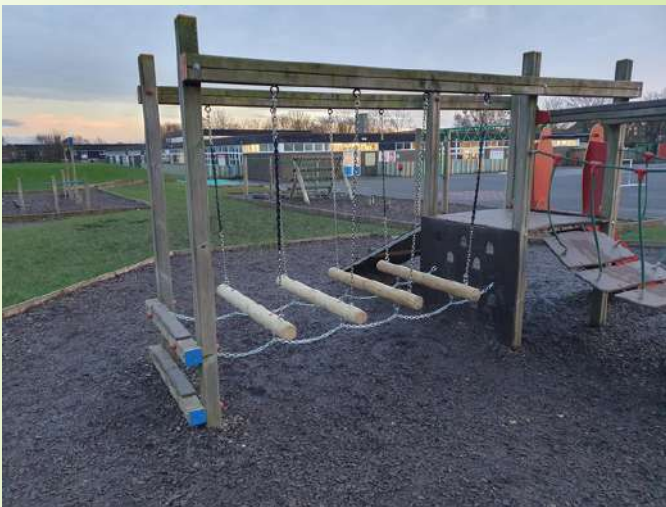
External Playground Equipment Repair. Primary School
