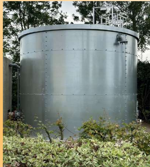
Replaced Sprinkler Tank Secondary School
