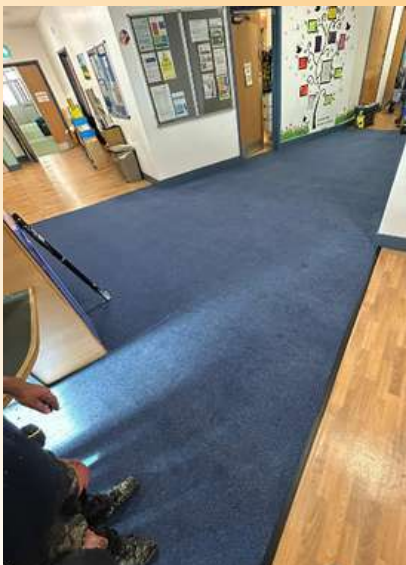
New Flooring Hospital - Lanchester
