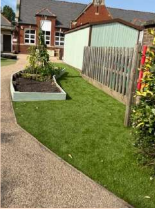
Artificial Turf Installation Primary School, Gateshead
