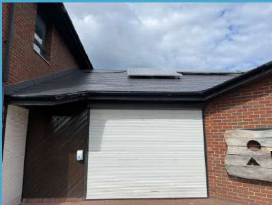
New guttering installed at a school.
