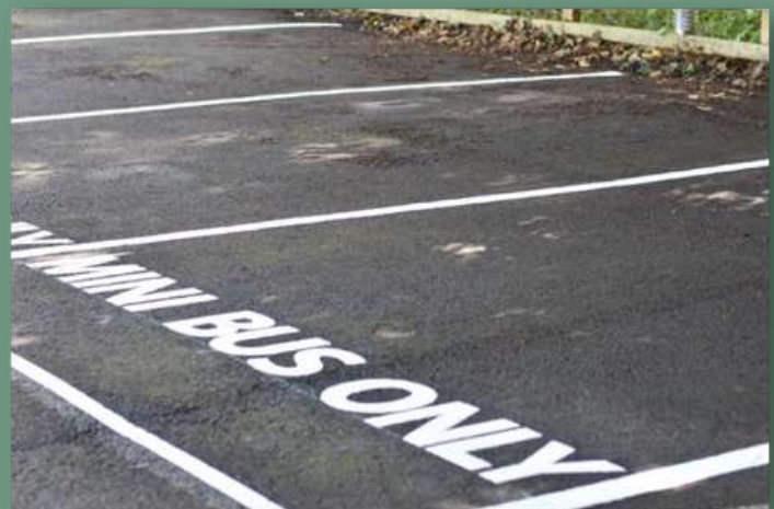
Creation & Painting of Car Park Markings. Primary School, Northumberland
