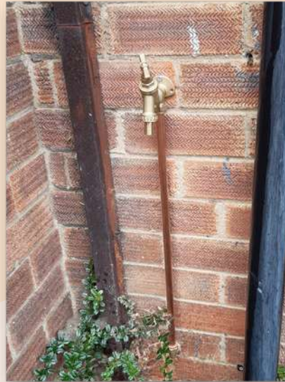
Installation of New Outdoor Tap. Newcastle
