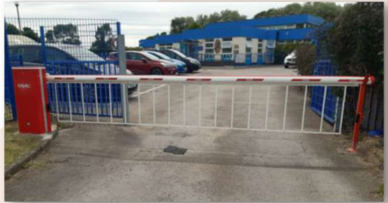
Installation of New Barrier. Secondary School. Northumberland
