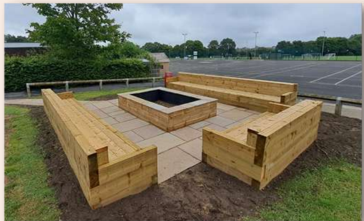
Design & Installation of Firepit. School, Ponteland
